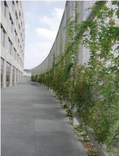
THE PREMIER AUTOMOTIVE GROUP FACILITY FEATURES 'GREEN' TRELLISES TO HELP INSULATE AND RETURN DISPLACED VEGETATION.
