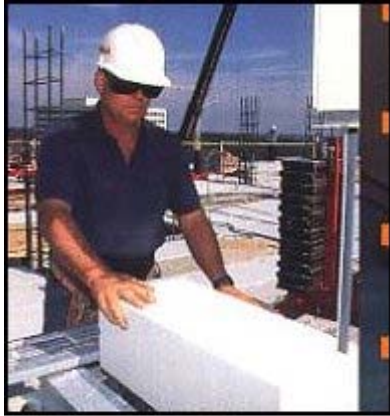
Autoclaved aerated concrete can be cut and shaped with wood-working tools.
