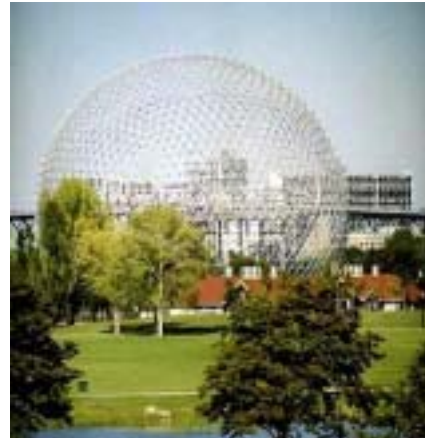
FIGURE 3.2b The geodesic dome of the U.S. Pavilion, Expo 67, Montreal protected the interior structures from sun, wind, and rain.
