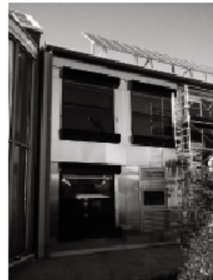
Fig. 1. View of the FASTEST site in Freiburg, showing four facade elements
