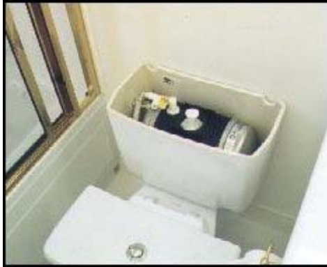
Storage tank inside toilet preserves city water pressure for flushing.
