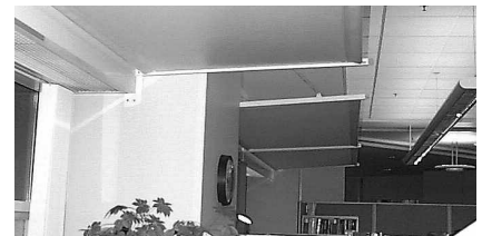
Figure 12: Sidelighting concept using stacked light shelves
