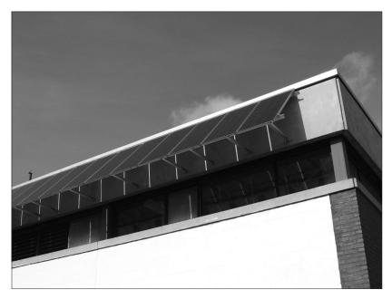
These photovoltaic cells are nicely integrated into an exterior building shading device.
