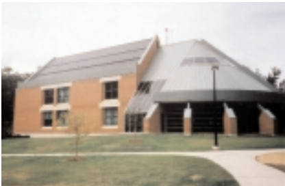
Figure 1: BIPV adds architectural distinction to roof components of this new building
