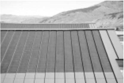
Figure 8: Example of standing seam roof
