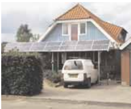
The other special mounting systems used in the SOL-300 project are (left) a newly-built pergola, and (right) a new extension using thin film solar cells.
