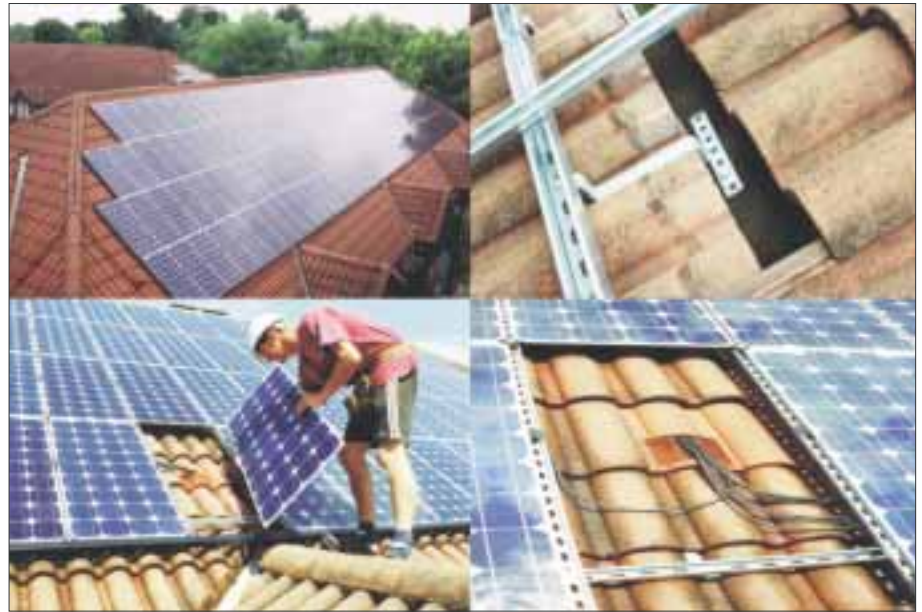
Installing the PV arrays on the Brockhill elderly residents home.
